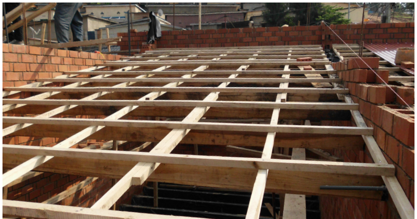
The roof structure completed with 6x4cm timber joists
