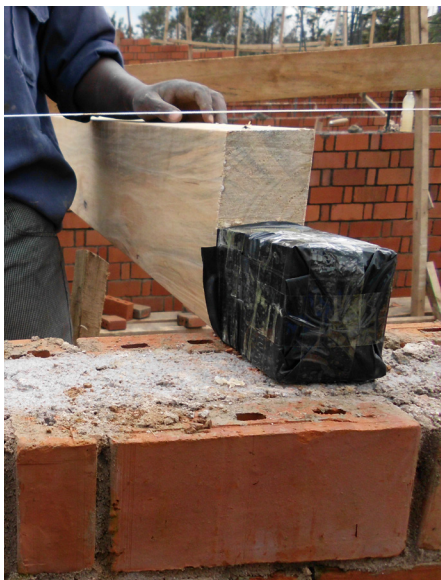
Waterproofed beam head
