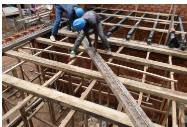
Maxspan rib being hoisted to position
