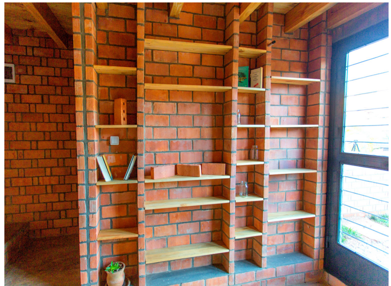
Interior 5,5x10x21cm brick partition wall with buttresses and in-built shelves
