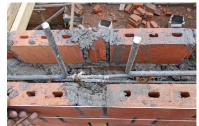
Tie beam waiting bars detail
