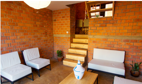
Example of RC + timber stairs connecting half/floor levels
