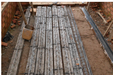
Maxspan ribs curing on site
