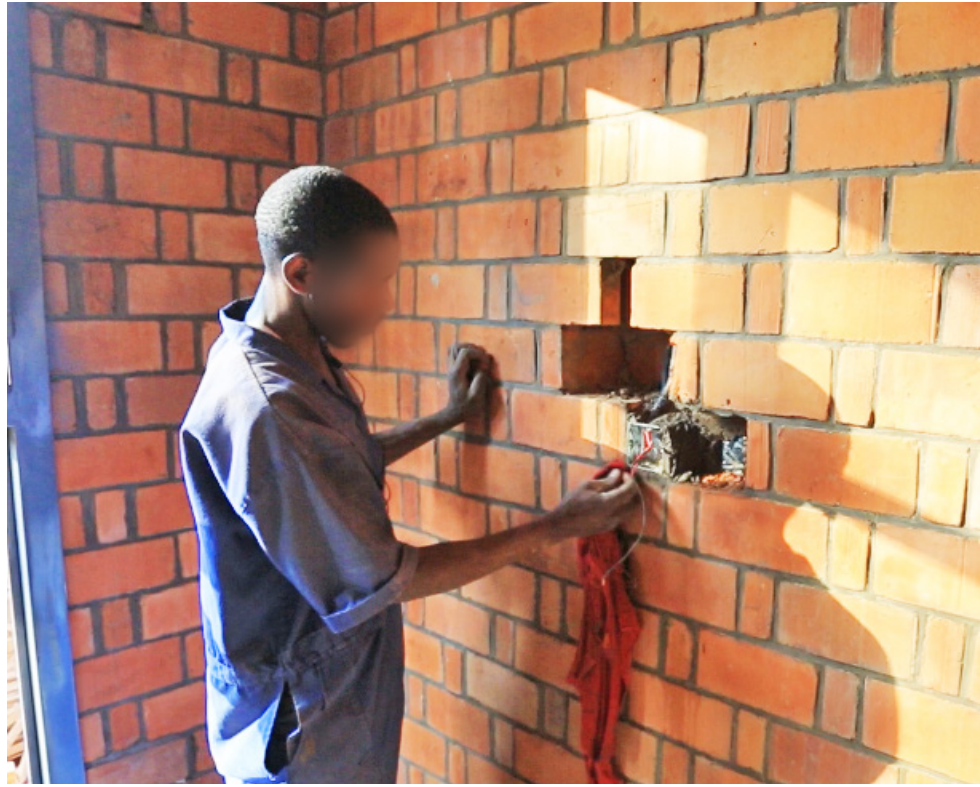
An electrician installing a light switch on a RLB masonry wall
