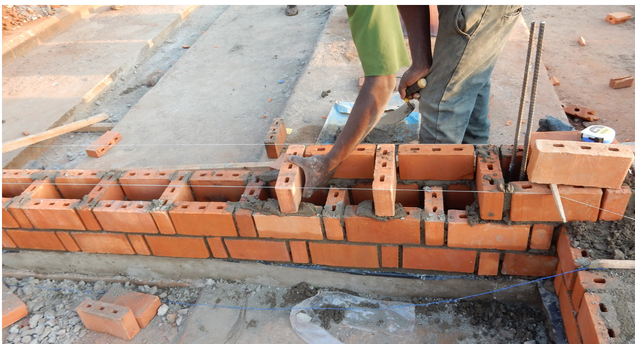
Row Lock Bond masonry wall construction
