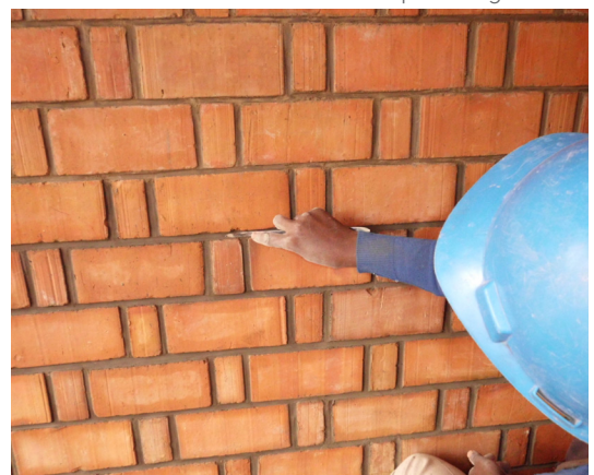
RLB wall cleaning works with water and vinegar
