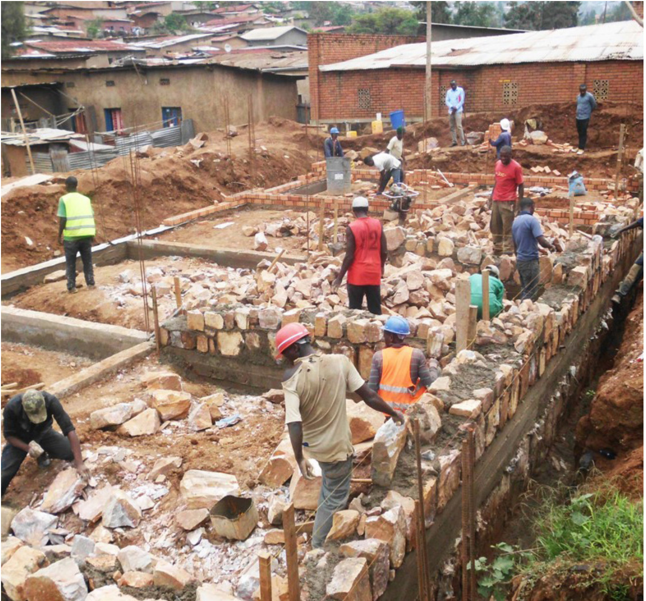
Construction of a stone masonry foundation wall.
