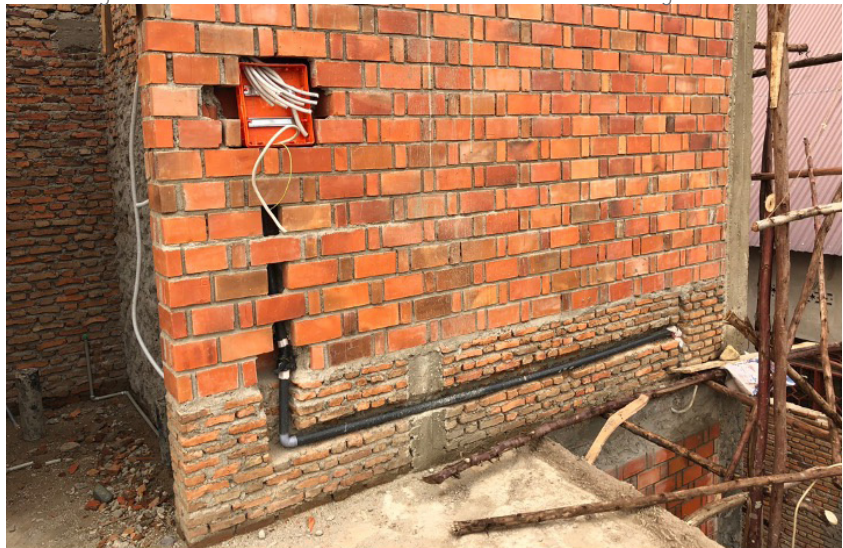
Mix of regular and RLB masonries and the different MEP integration solutions
