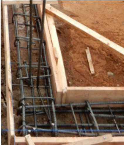
Typical ground beam reinforcement.
