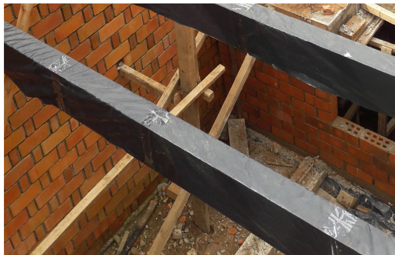
Detail view of the timber beam and RLB wall connection.
