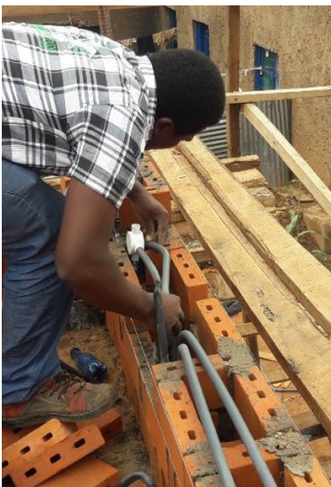
An electrician working on conduits installation within the RLB cavities
