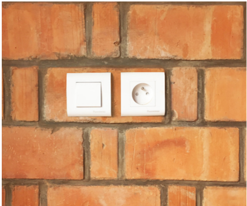
Sockets and switches installed on a RLB masonry wall
