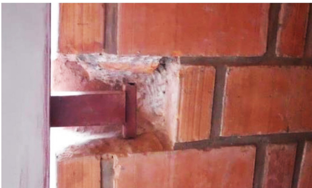
Frame bracket positioned within the brick wall pattern
