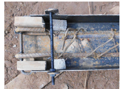
Pre-cast beam nose end detail
