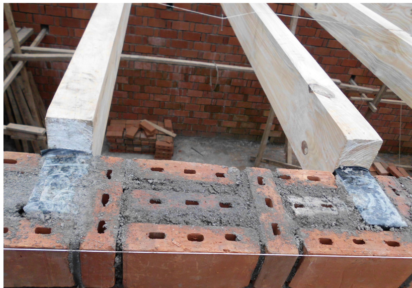
Detail view of the timber beam and RLB wall connection.
