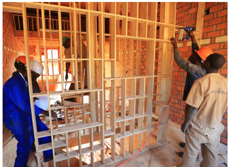
Timber frame partition under construction
