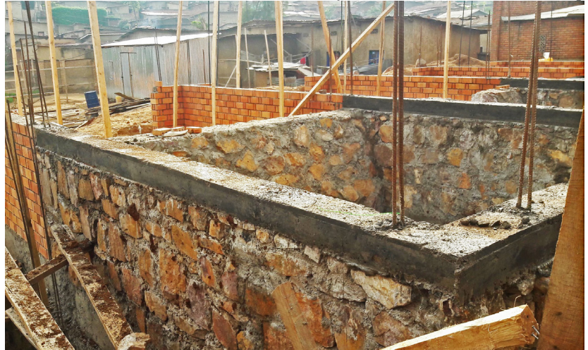
Ground beam and stone masonry foundation before backfilling
