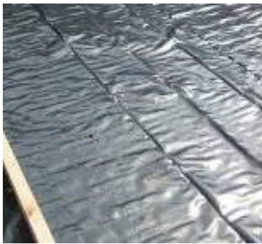
Damp proof membrane laid over the hardcore layer
