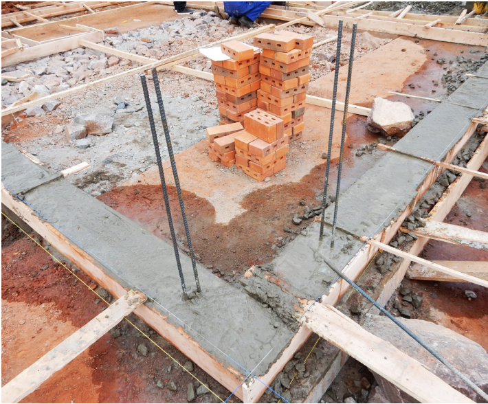
Ground beam and vertical waiting re-bars.
