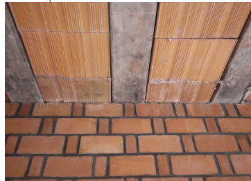
Maxspan bare slab underside
