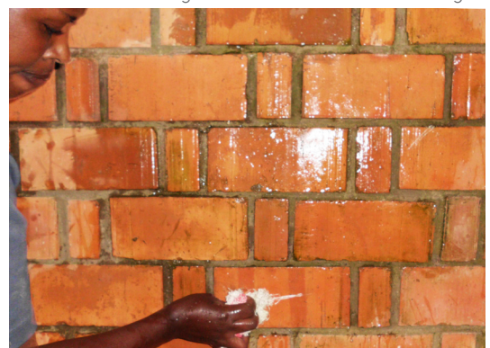
RLB wall cleaning works with water and vinegar
