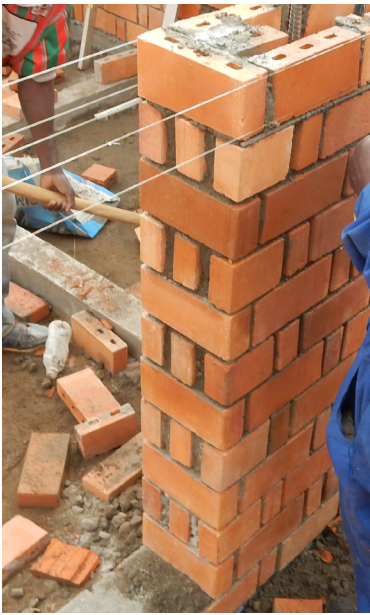
RLB wall side before a door installation
