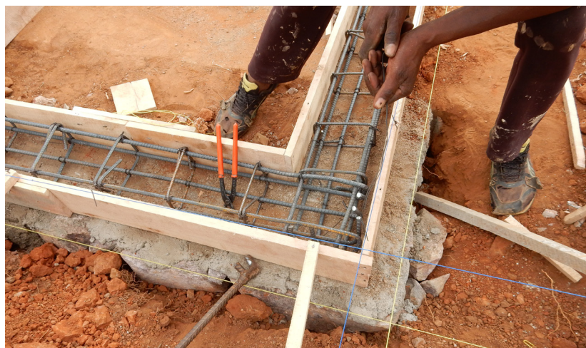
Examples of a plinth beam reinforcement cage.
