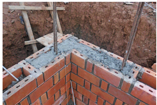
Corner reinforced concrete tie beam
