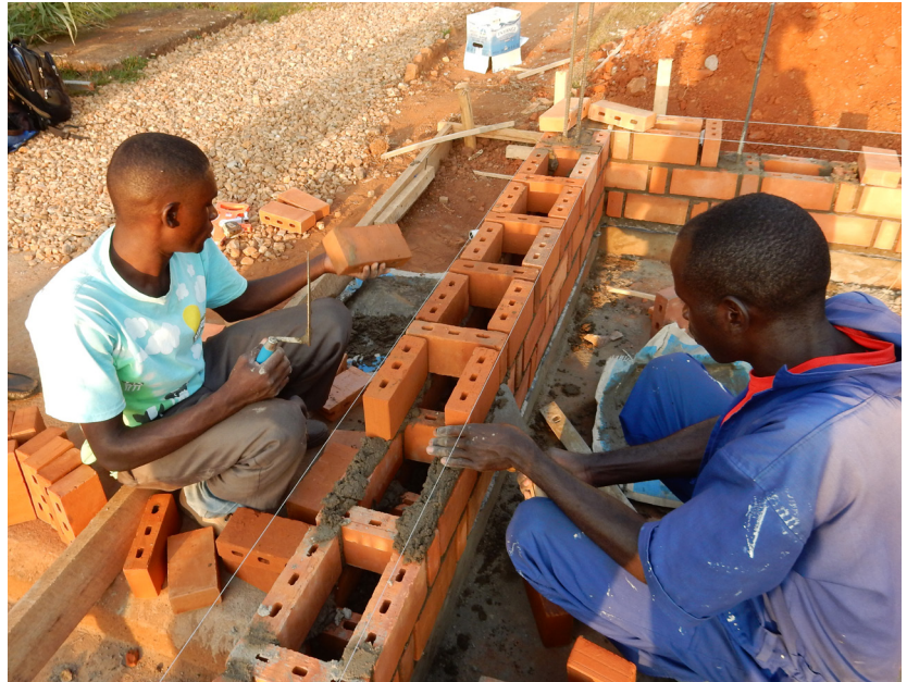
Row Lock Bond masonry wall construction
