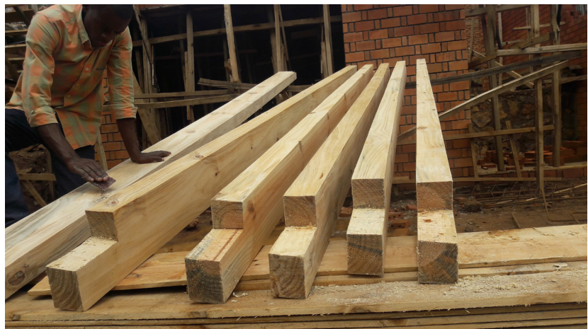
Timber beams being sanded and treated before the installation
