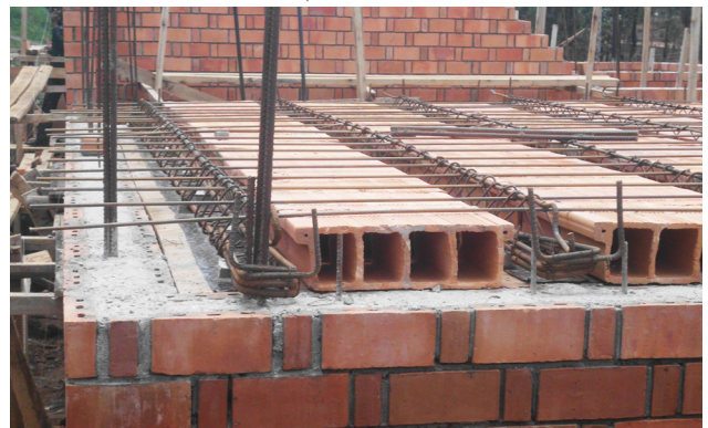
Detail of the in-situ Maxspan ribs reinforcement and blocks
