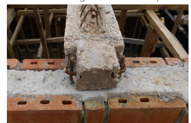
Maxspan/tie beam connection detail
