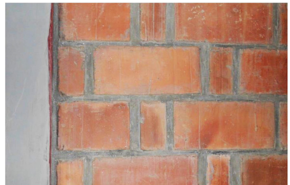
Masonry completed and pointed
