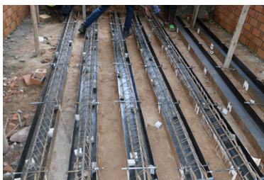
Maxspan ribs formworks
