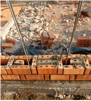
Rebars protruding from the ground beam and the RLB masonry
