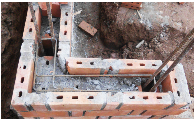
Corner reinforcement bars connecting with the columns.
