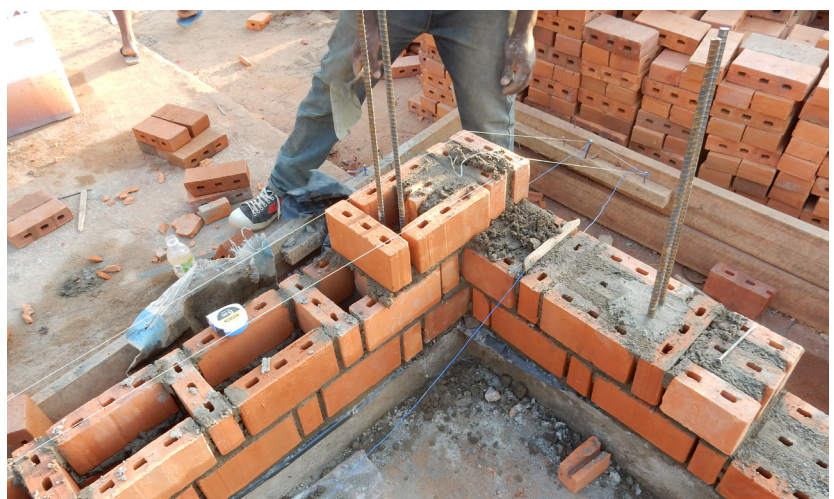
RLB wall intersection reinforcement
