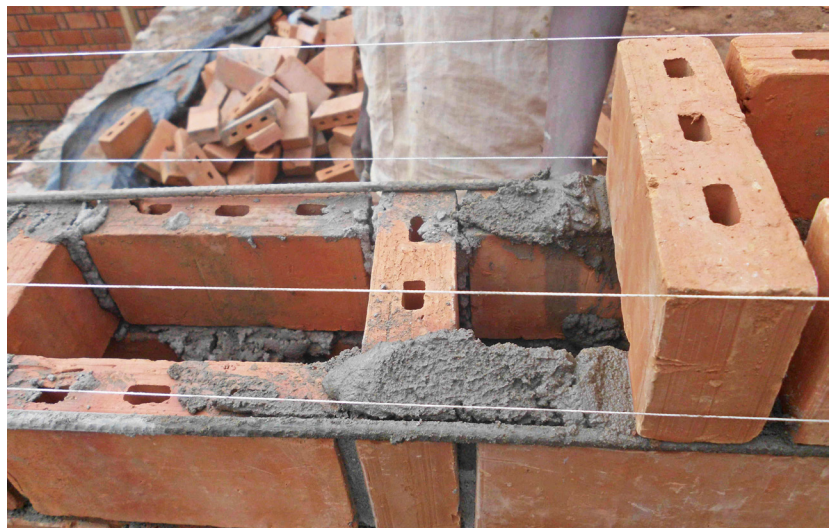
Re-bar used as gauge to control the joint thickness and alignment strings
