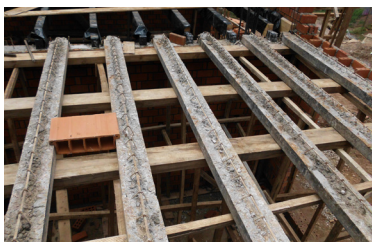
Maxspan blocks placed in-between ribs
