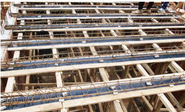
In-situ Maxspan rib reinforcements positioned over the formwork
