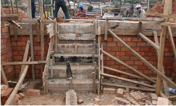
Example of RC + timber stairs connecting half/floor levels
