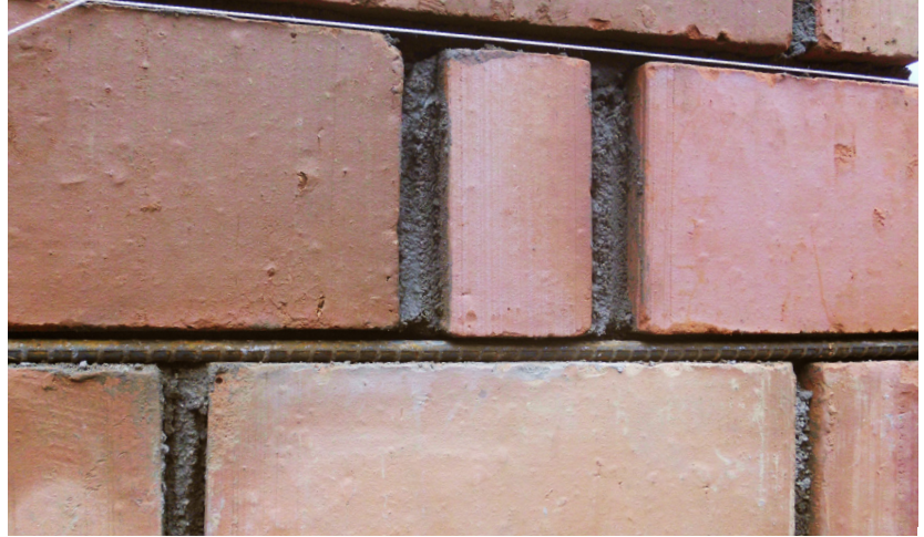
Re-bar used as gauge to control the joint thickness
