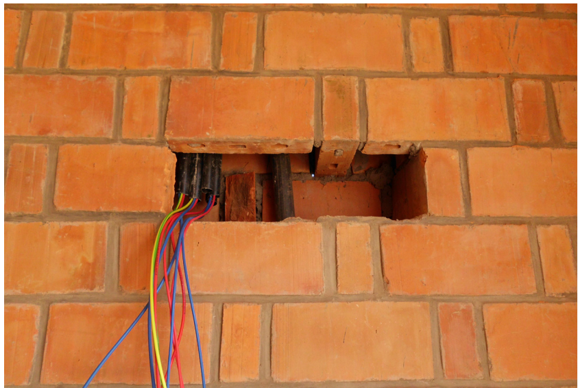
Electrical conduits and cables routed through the RLB cavities
