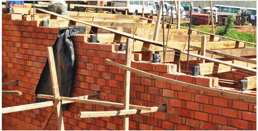
Roof timber beams in position before the wall construction continues
