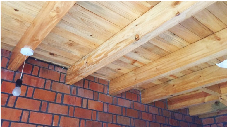
A suspended Pinus beams and Pinus T&G planks floor
