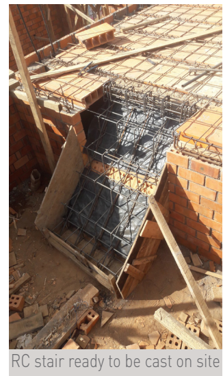
RC stair reinforcement diagram
