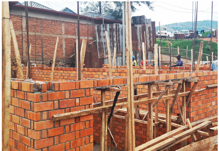
A typical RLB masonry elevation with doors and windows of different sizes
