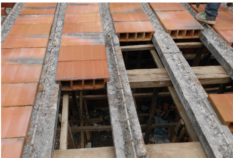
↑ Maxspan blocks placed in-between ribs
