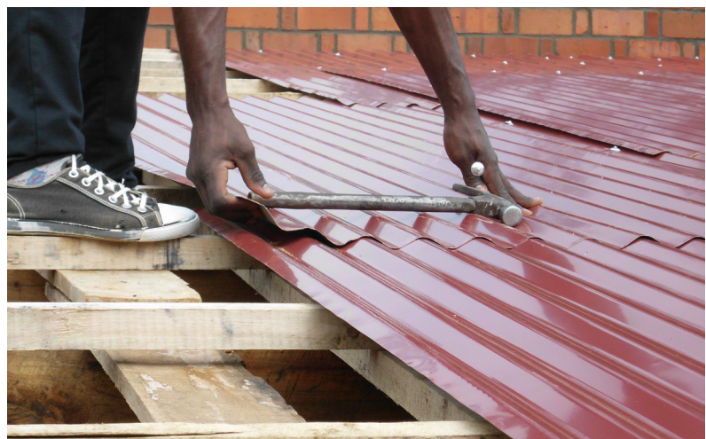
Corrugated metal sheets installed with a minimum 15cm overlap
