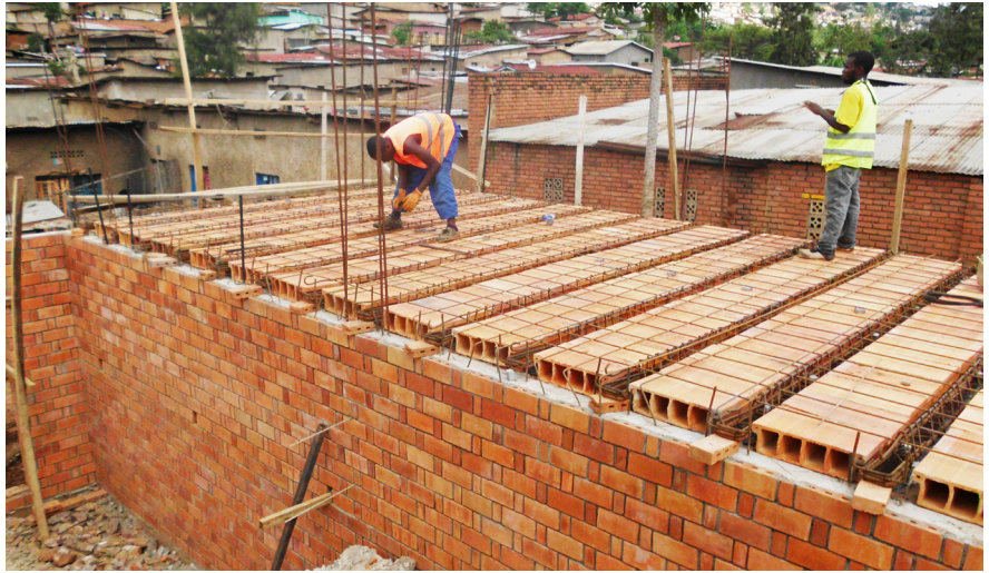
In-situ Maxspan in the works
